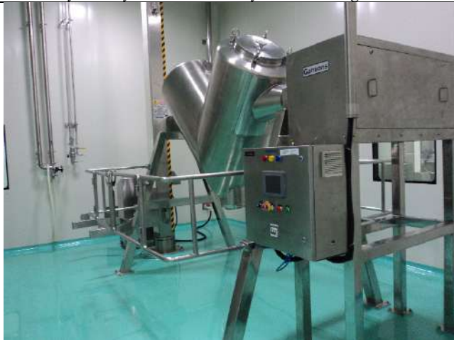
Supplied, installed, commissioned and calibrated manufacturing equipment along with utility equipment
