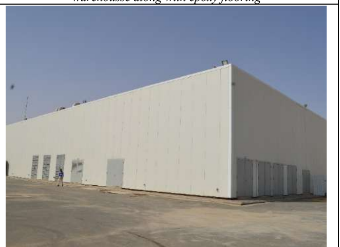
Exterior view of the facility
