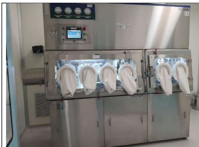
Supplied, installed, commissioned and calibrated dispensing isolator
