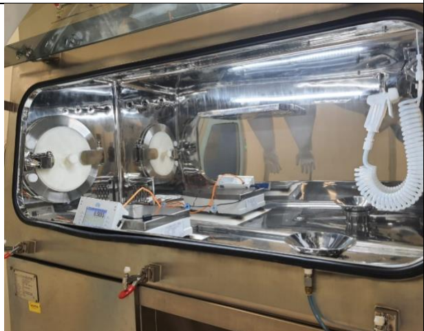
Supplied, installed, commissioned and calibrated sampling isolator
