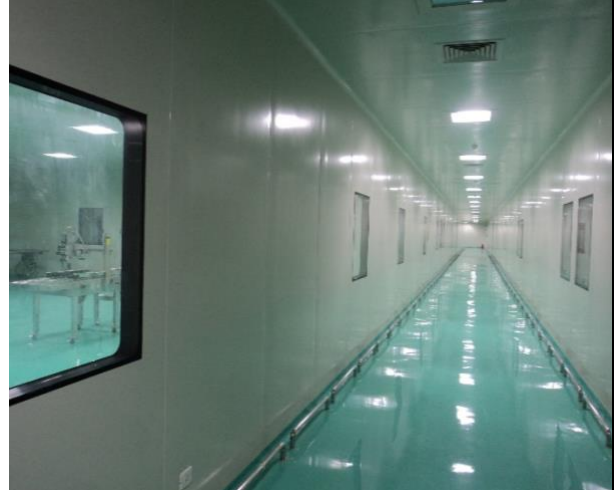
Facility corridor where cleanroom walls, ceiling and view panels have been installed along with epoxy flooring
