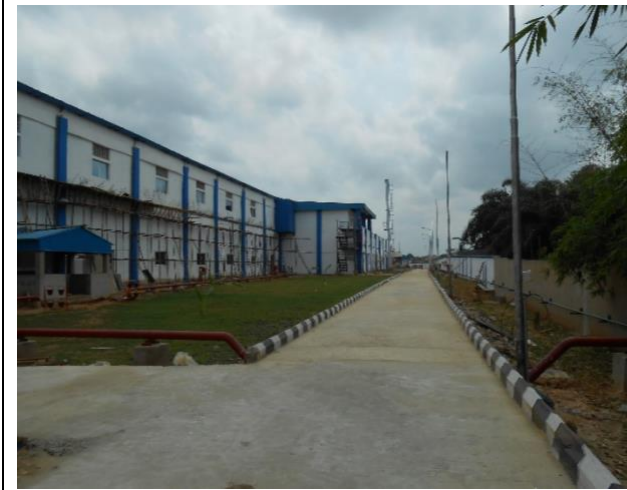
Exterior facility with pre-engineered building structure, fire hydrant system, raw water system, street light etc.
