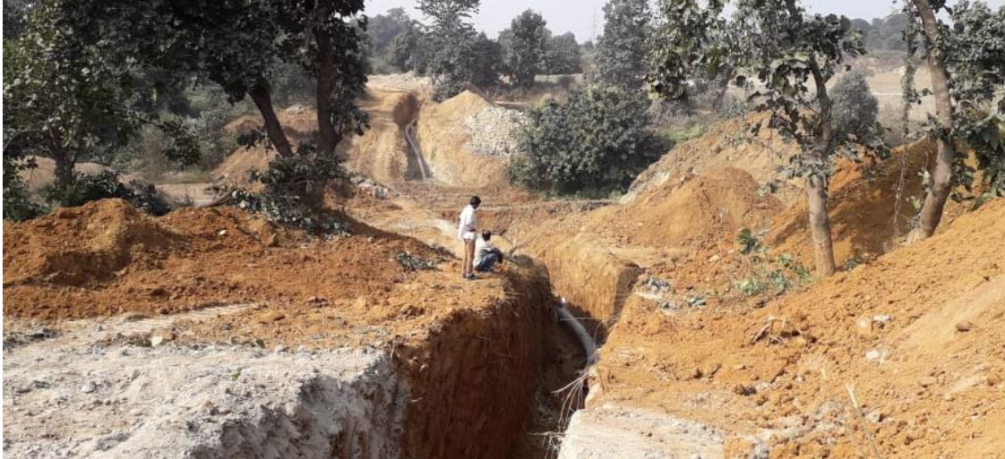
Pipeline laid for a Cross-Country Project
